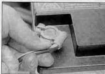
C Check the security and condition of the battery terminals.
