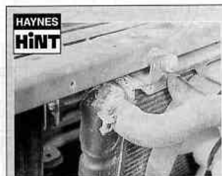
A leak in the cooling system will usually show up as white or rust coloured deposits on the area adjoining the leak.
