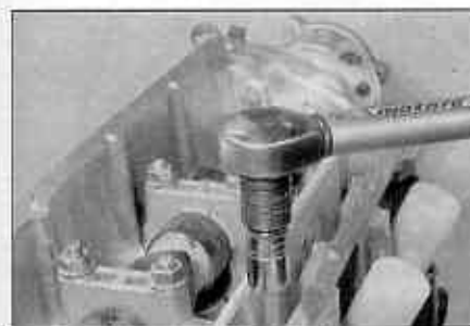
9.52b Tighten the cylinder head bolts to the Stage 1 and Stage 2 settings using a torque wrench
