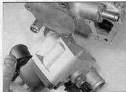
4.6c Removing the thermostat housing (diesel engine)
