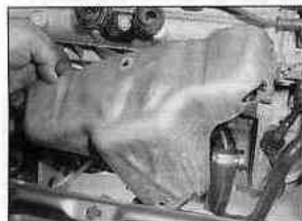
5.5a On 16-valve engines, undo the bolts and remove the manifold heat shield . . .
