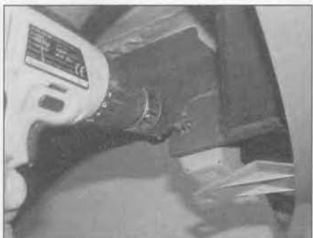
28.19a Drill a 12.5 mm diameter hole through the bumper mounting brackets each side ...
