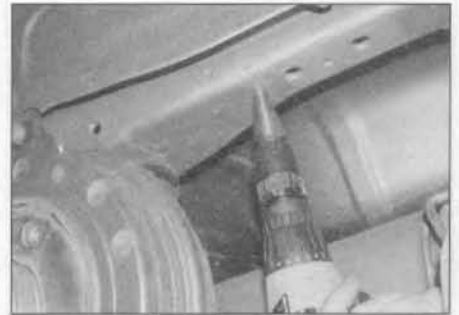
28.12a Drill a pilot hole at the position marked, then enlarge the hole using a conical hole cutter . . .
