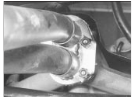
44.15 Exhaust downpipe flange nuts
